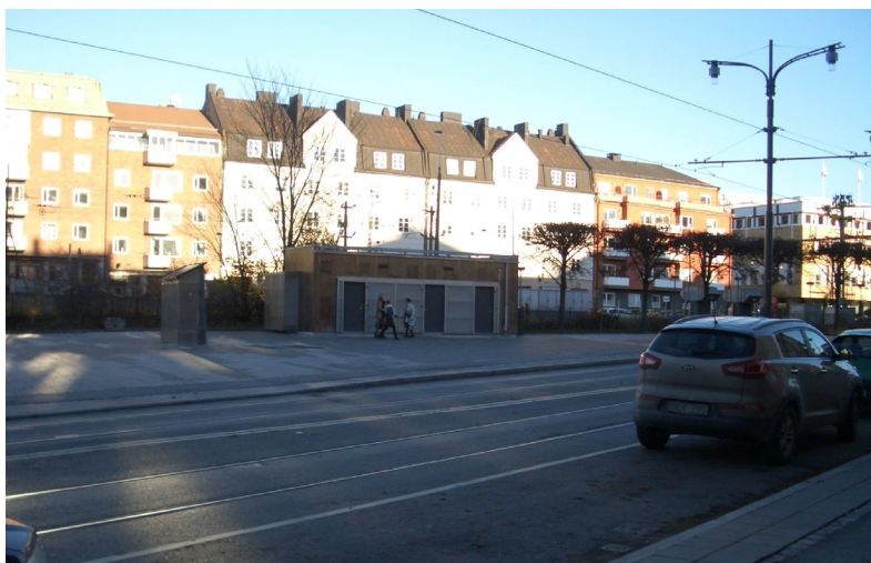
Omformerstation i Stockholm
